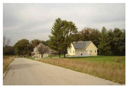
Homes at <u>Sugar Creek Preserve</u>. The lack of curbs and gutters on narrow roads allows storm water to infiltrate natural lands, recharging groundwater instead of polluting area lakes and streams, to preserve clean water, and to save municipalities storm water pollution treatment costs.
