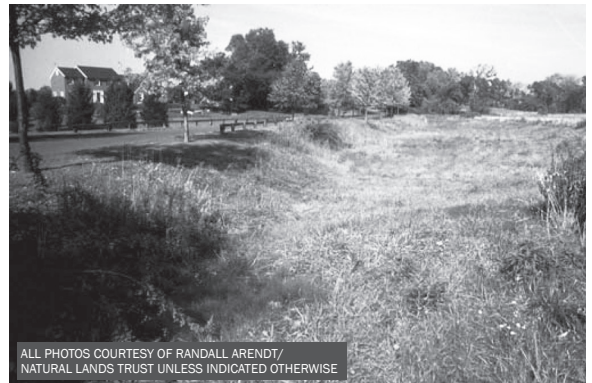
Infiltration or conservation meadows are a less expensive and environmentally superior alternative to deep “bomb-crater” basin designs. In this example from Doylestown Township in Bucks County, the side slopes are so gentle that the entire meadow can be mowed with large equipment once a year, saving the township money and manpower. It also provides habitat for birds, insects, bats, and other small mammals.
