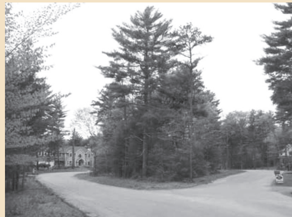
When the boulevard model is not feasible, cul-de-sacs should at least include an island planted with canopy shade trees to properly fill the space in the center of this bulbous street form. Existing trees could also be left in place in the center. Plowing snow is much easier in such a design because plow operators can make one efficient sweep around the central island.
